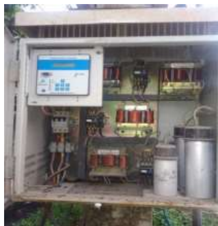
Figure 22. APFC Panel and Energy Meter connected at pole
