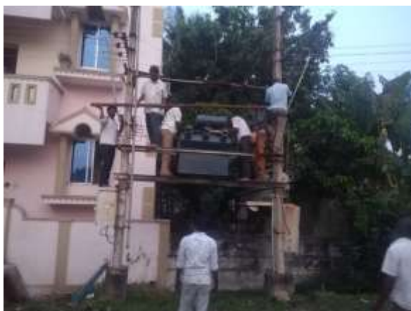
Figure 21. Connecting Active Repaired DT back into the DT at Chengalpet Electricity Distribution Circle
