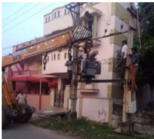
Figure 20. Removing existing DT for replacing it with Active Repaired DT
